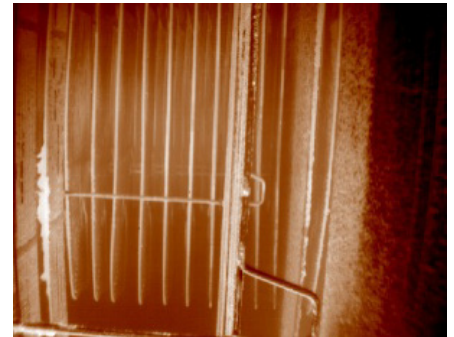
Superheat pendants in 700MW power boiler burning PRB coal
